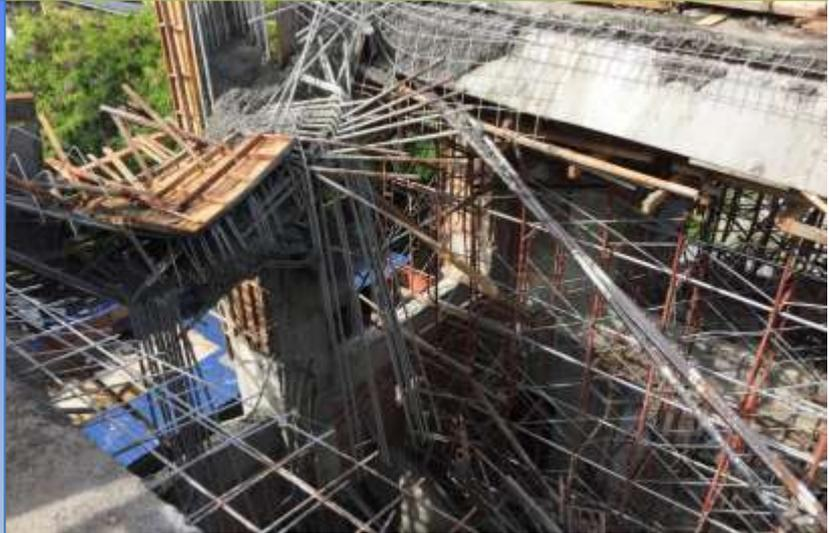
A falsework collapsed during concreting works in construction site in Kuala Lumpur. The accident causing 1 worker died. Based on investigation, cause of the accident was the falsework structure not capable to bear the applied load. Lack of co-ordination between the contractors, engineers and suppliers of falsework material and lack of understanding on structural shoring details and requirements could possibly be the underlying cause of the accident.
