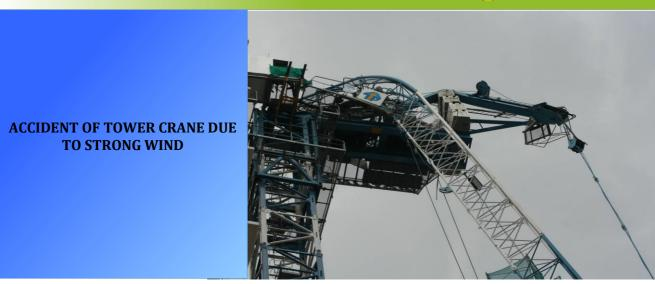
Recently, an accident had occurred involving parked tower crane. The incident occurred on Sunday due to strong winds when the crane was not in the operation. The investigations found the crane failed to slew during the strong wind and caused very high load on the boom structure and subsequently fell to the adjacent building. Hence, these steps should be followed to avoid the same occurrence:
