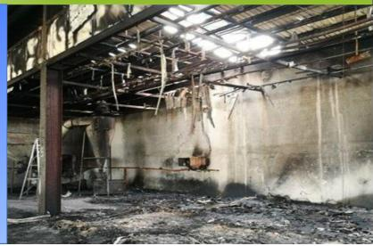
On October 2, 2016, a dust explosion has occurred in the kenaf processing plant. These kenaf stem are burnt out to produce final product as a charcoal. The explosion has been affected to the processing area and caused serious injury to the worker and defects to the building.
