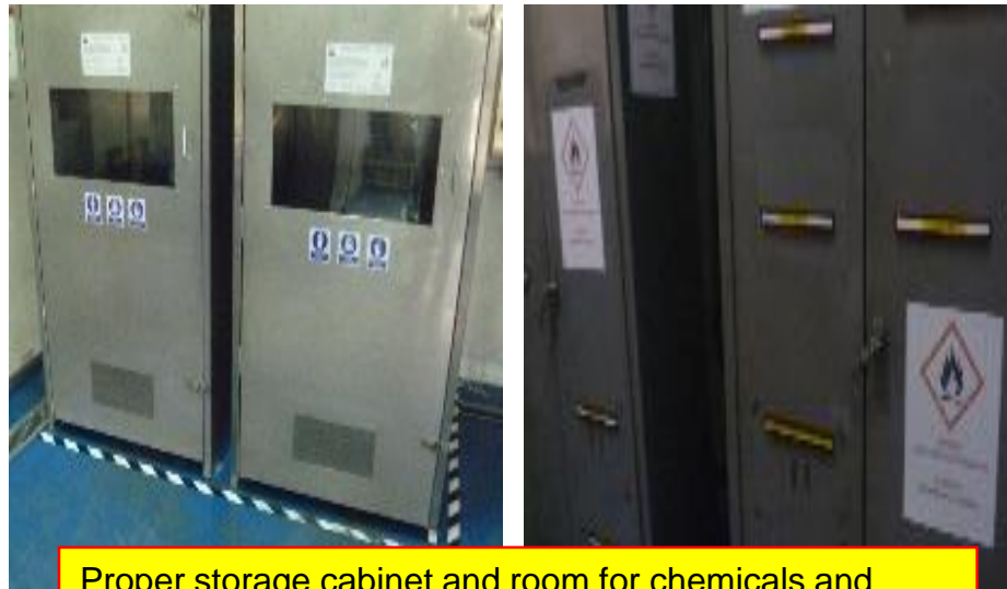
Proper storage cabinet and room for chemicals and automated dispensing system
