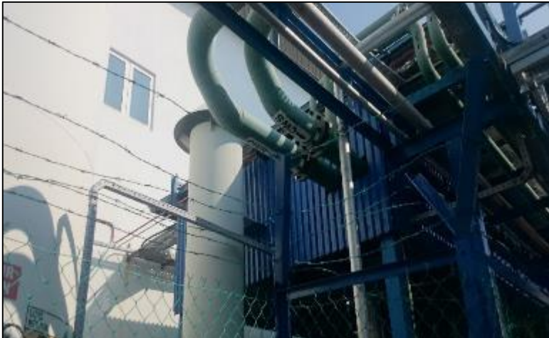
Install sound proof equipment & building windows for the N2 plant area which is adjacent to the building(<80dB)
