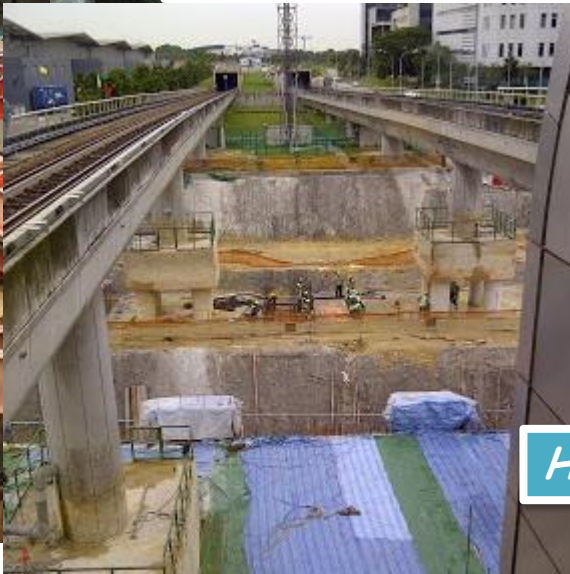
Underpinning Works / Works under Existing Railway
