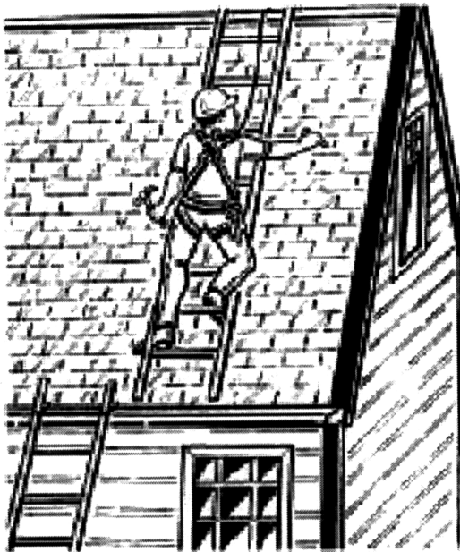
Fig. 18 Bracket on roof ladder should reach over the ridge
