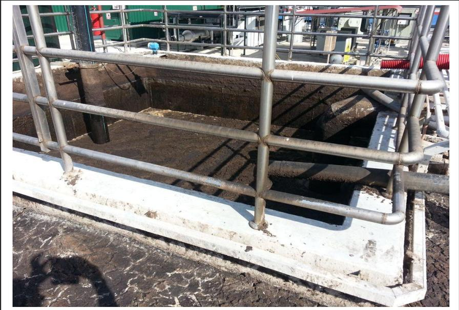
*Figure 7: Under Ground Mixing Pit (Source: FGV)*
