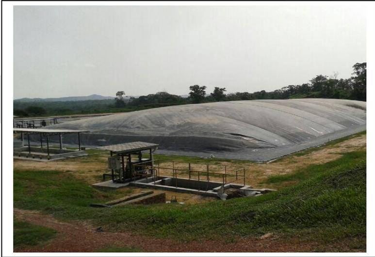
A wide-angle photograph of a large, white, dome-shaped anaerobic digester pond. The pond is situated in an open field with some concrete structures and a small building in the foreground. The background shows a line of trees and a clear sky.</div> <p data-bbox="674 1366 1283 1404"><i>Figure 11: CA digester pond (Source: FGV)</i></p> |         |
