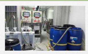
Installed extended hose system & location - No transferring of drum & turning needed
