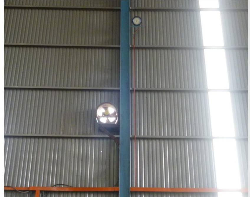
Workshop fitted with ventilation system fan
