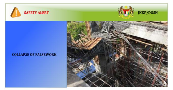
A falsework collapsed during concreting works in construction site in Kuala Lumpur. The accident causing 1 worker died. Based on investigation, cause of the accident was the falsework structure not capable to bear the applied load. Lack of co-ordination between the contractors, engineers and suppliers of falsework material and lack of understanding on structural shoring details and requirements could possibly be the underlying cause of the accident.
