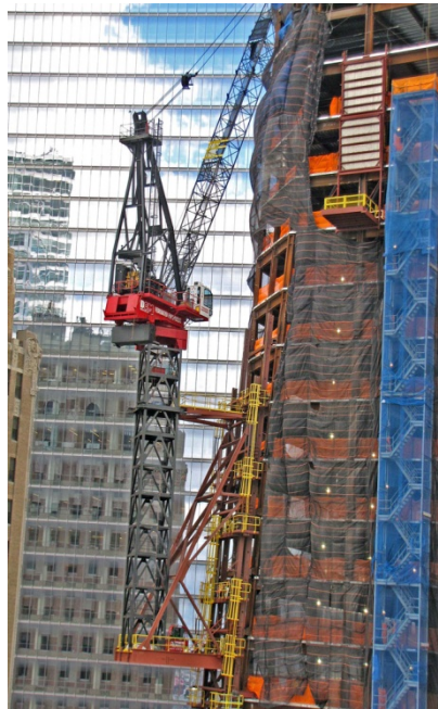
Figure 2.11 Installation of crane with external climbing base ( www.dcm.milgromandassociates.com )
