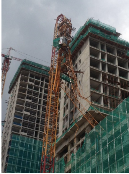
Figure 6.6 Condition of the tower crane after the incident
