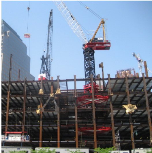
Figure 2.12 Installation of a crane with an internal climbing base ( www.dcm.milgromandassociates.com )
