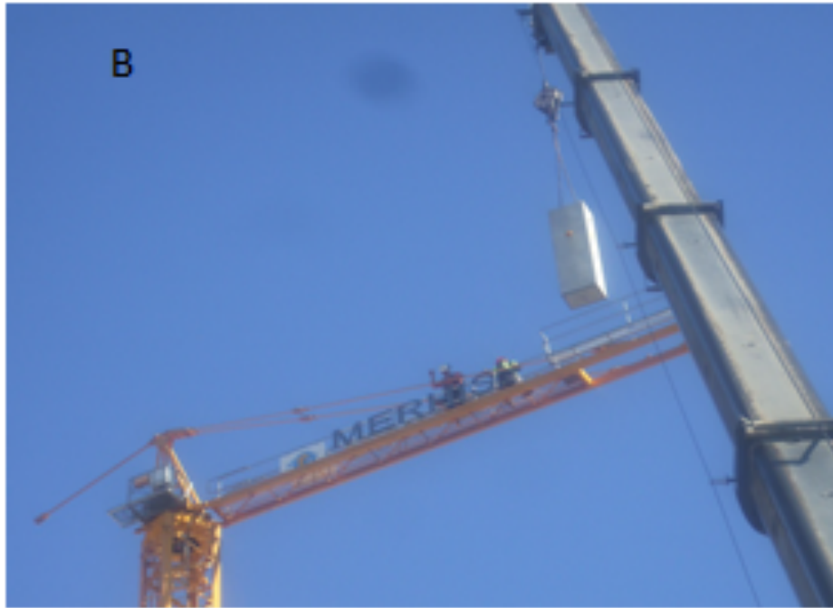
Figure 10.6 Methods of dismantling the counter weight
