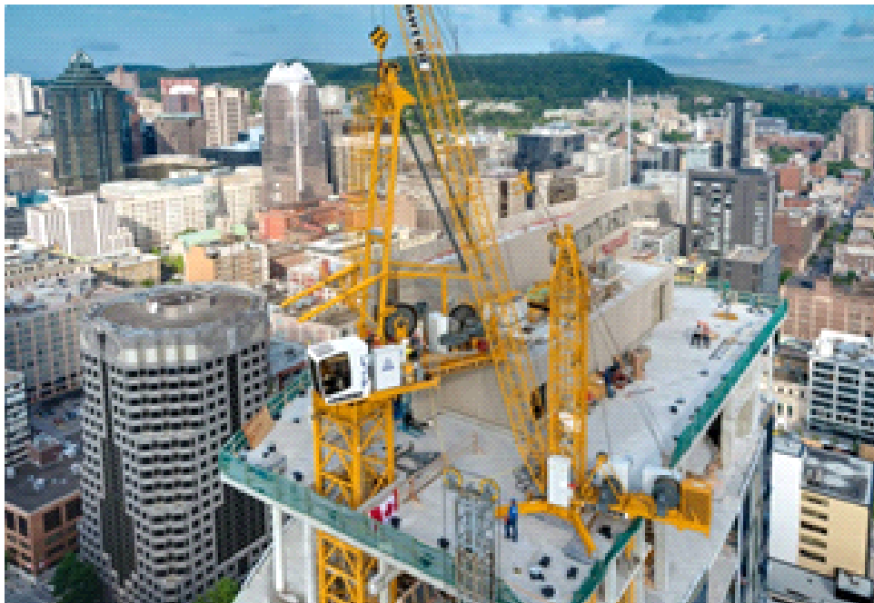
Figure 10.12 Derrick crane for tower crane dismantling work
