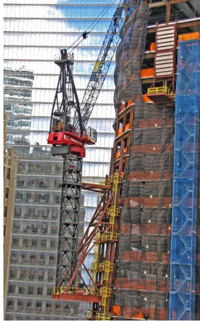
Figure 2.11 Installation of crane with external climbing base ( www.dcm.milgromandassociates.com )
