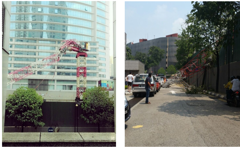
Figure 10.6 Luffing tower crane accident in Bangsar
