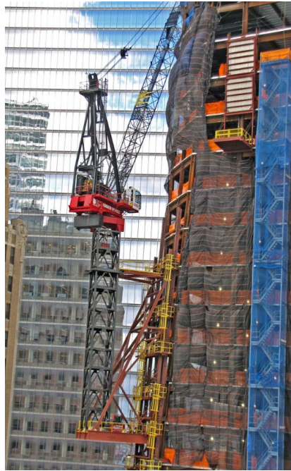
Rajah 4.7 Installation of crane with external supported static crane ( www.dcm.milgromandassociates.com )
