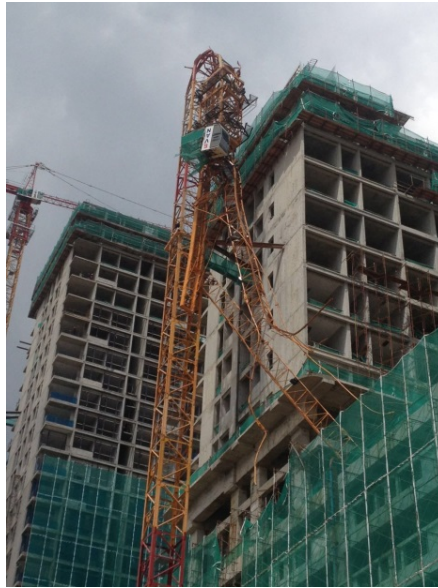
Figure 10.7 Condition of the tower crane after the incident
