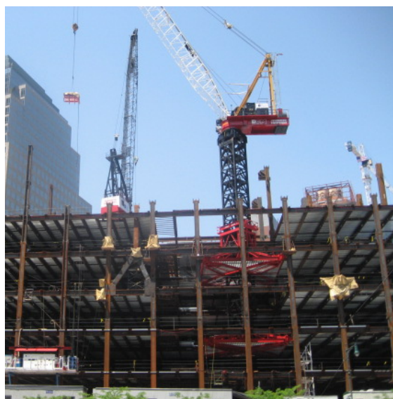
Figure 4.8 Installation of crane with internal climbing crane ( www.dcm.milgromandassociates.com )
