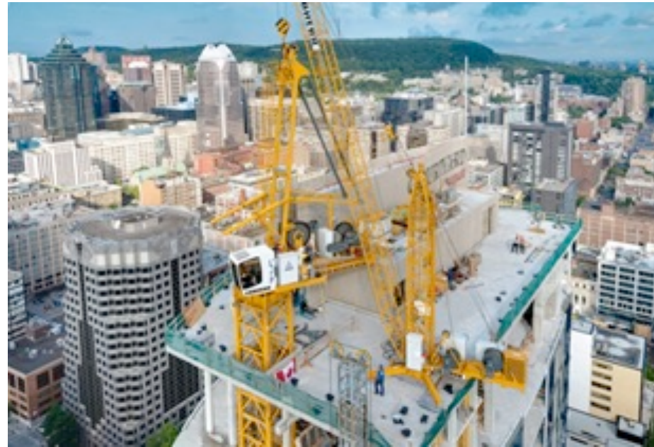
Derrick crane for tower crane dismantling work
