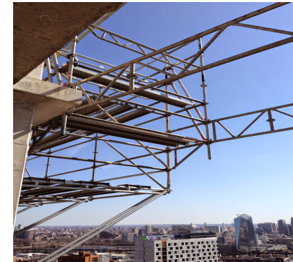
Cantilevered temporary work platforms
