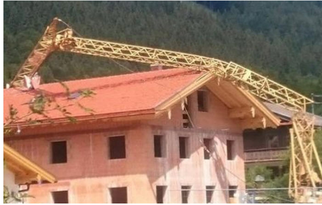
Figure 2.34 Tower crane accident in Bavaria due to metal fatigue failure at the jib support ( http://www.craneaccidents.com )
