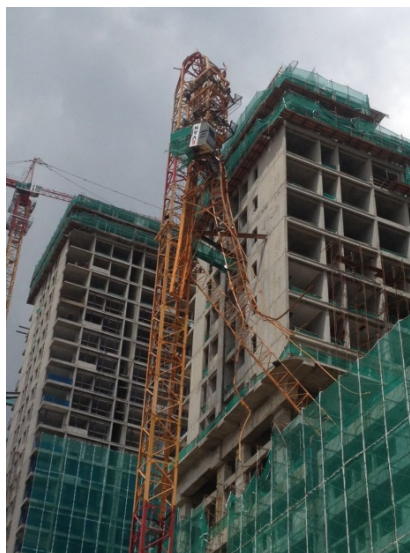
Figure 4.11 The snapped crane happen at Johor (2016)
