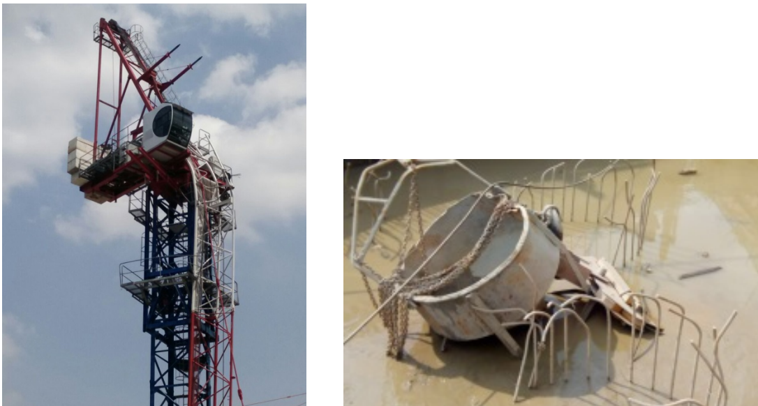
Figure 4.10 Failure of crane in Jelatek (a) The broken crane, (b) used bucket stuck on crag
