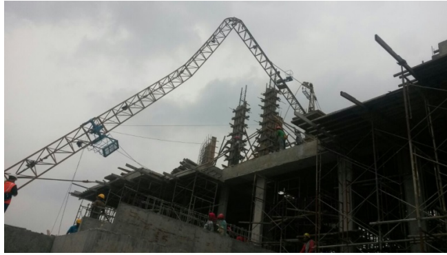
Figure 4.12 Bent crane boom
