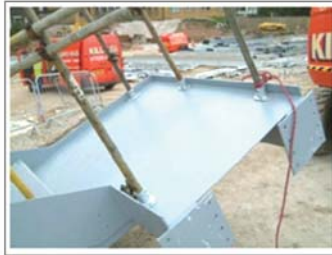
Temporary stair handrails installed at ground level (same holes were later used for the permanent handrail)
