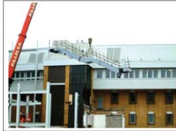
Staircase with Edge Protection being lifted into the Structural Steel Frame
