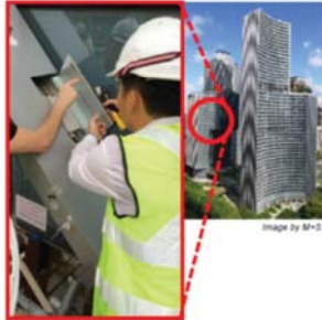
Facade lighting fixtures should be easy to access for maintenance
