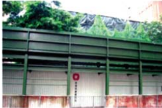
Double deck hoarding / covered walkway to protect pedestrians; locations and extent of hoarding should be clearly defined
