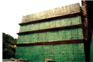
Scaffold, nylon mesh and periphery catch platforms / fans to prevent demolished debris from falling out of the block
