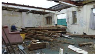
Demolition was carried out by hand with workers climbing on to the unguarded roof. Image: HSE
