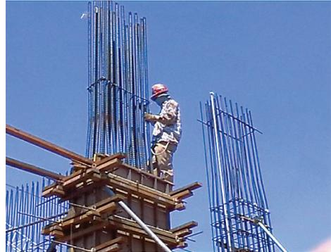
20.4.2 The formwork including the shores, braces and other supports shall be inspected by the designated person:-
