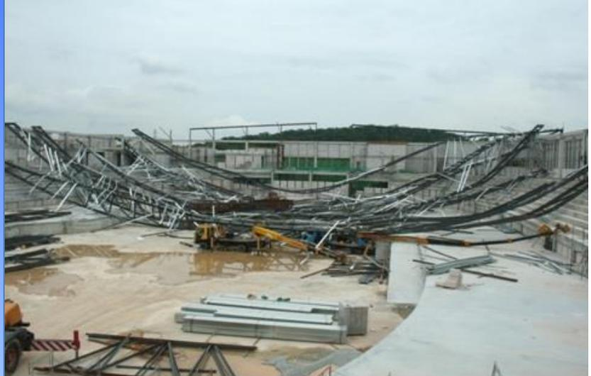
An incident involving the collapse of a roof truss structure which is in the process of installation in a velodrome has occurred at approximately 3:00 pm, June 18, 2016 in Nilai, N.Sembilan. Two skylift machinery under the roof structure has been crushed by the collapsed roof structure. The skylift machinery was used to lift workers to do the connection work on roof structure. This incident also caused a worker injured and no casualties occurred.
