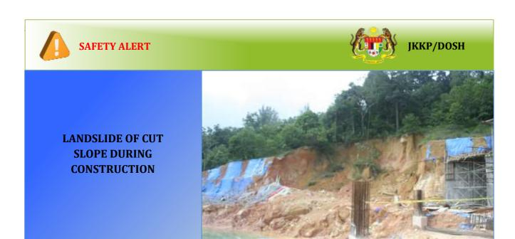
Accidents involving slope landslide have occurred at a construction site which has resulted in eleven workers killed while they are working nearby the slope's toe. Prior to the incident, slope stabilization work is in progress and at the same time with construction work which is also carried out in the area radius of slope.
