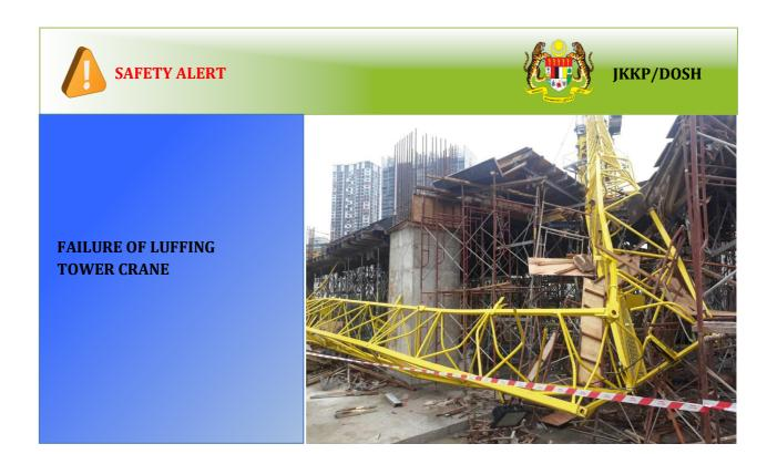
A accident involving a luffing tower crane had occurred in a construction site. In the accident, the structure of the boom fall and broke. The boom hit four workers. The four workers were installing the formwork at the first floor. During the accident, no load were carried by the crane. It occurred at about 10.40 am, where one worker was death and three workers were injured.
