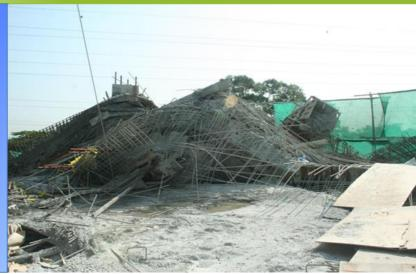
A falsework collapsed during concreting works in construction site in Petaling Jaya. The accident causing 1 worker died and 5 others injured. Cause of the accident was the structure not capable to bear the applied load. Lack of co-ordination between the contractors, engineers and suppliers of falsework and erectors lack of understanding on structural shoring details and requirements maybe the underlying cause of the accident.
