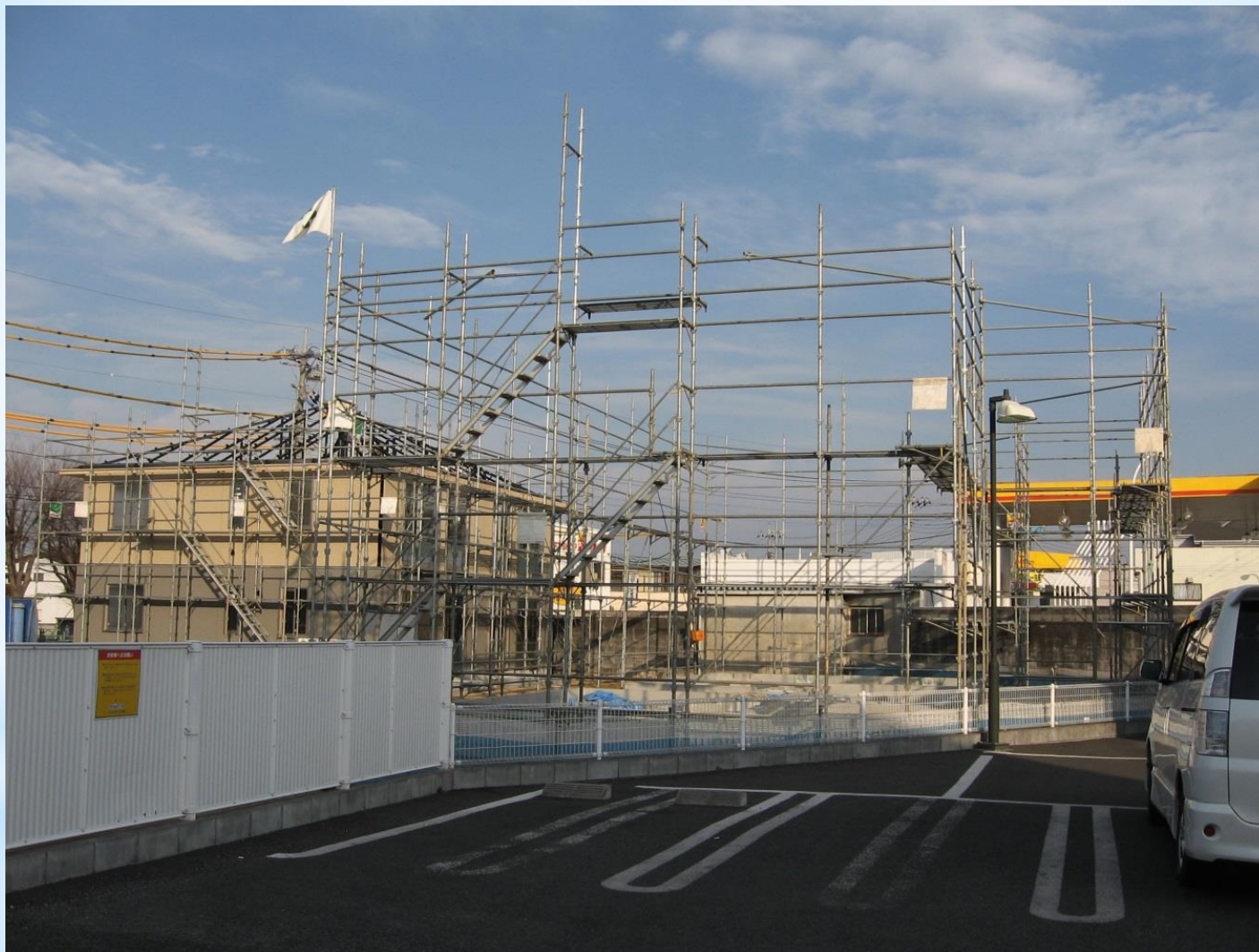
Methods to Erect Scaffolds First for low-rise house construction (Height of a house is less than 10m)
