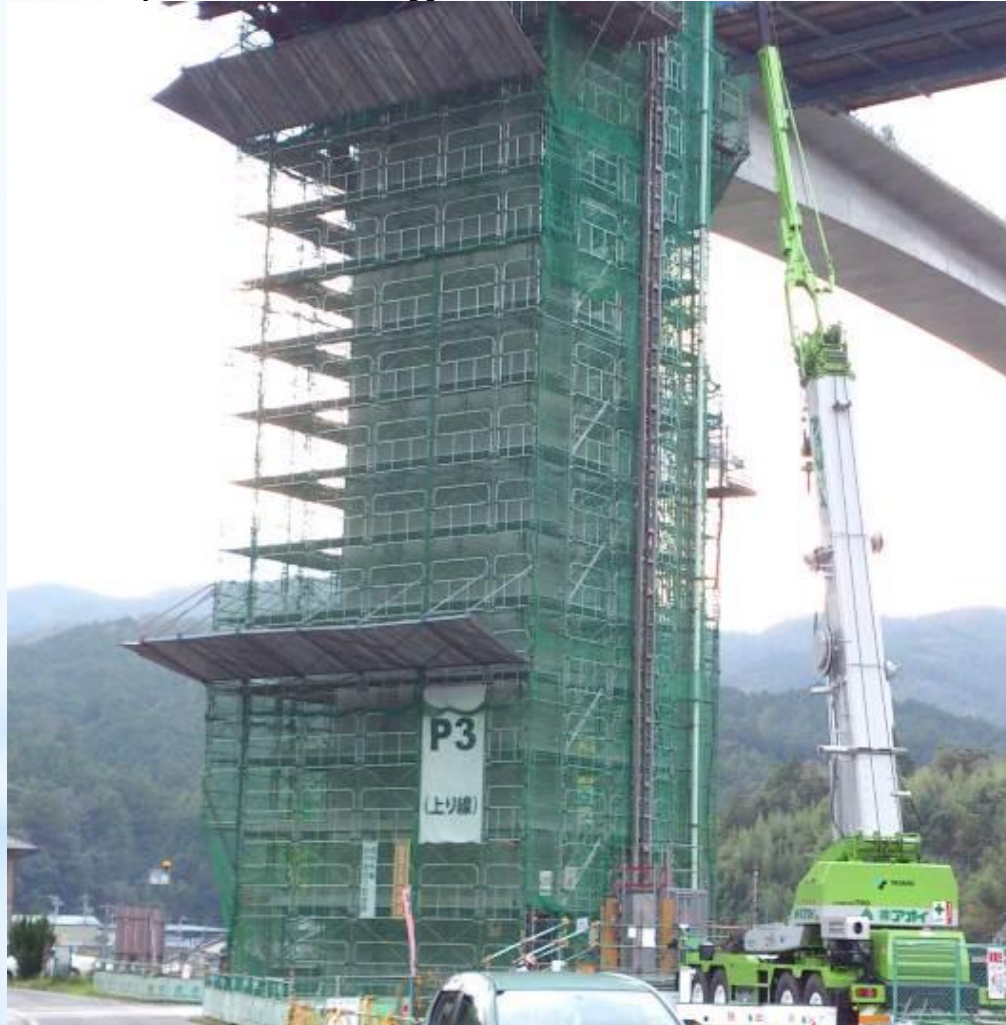
Scaffolds assembled by Methods to Erect Handrails First
