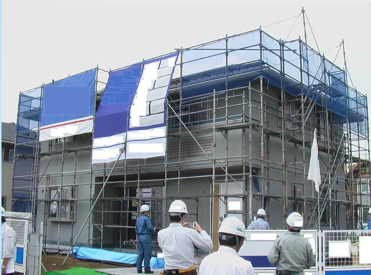
A house constructed by Methods to Erect Scaffolds First
