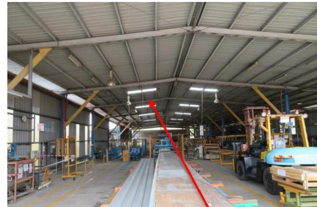
Factory B – Rear of factory's roofing panel replaced with translucent roofing sheet.
