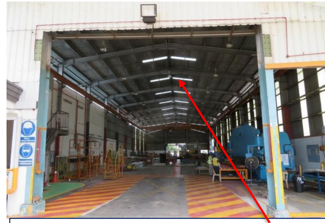
Factory A – Alternate roofing panel replaced with translucent roofing sheet.
