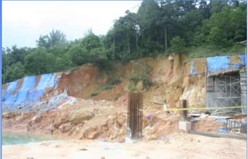
Accidents involving slope landslide have occurred at a construction site which has resulted in eleven workers killed while they are working nearby the slope's toe. Prior to the incident, slope stabilization work is in progress and at the same time with construction work which is also carried out in the area radius of slope.
