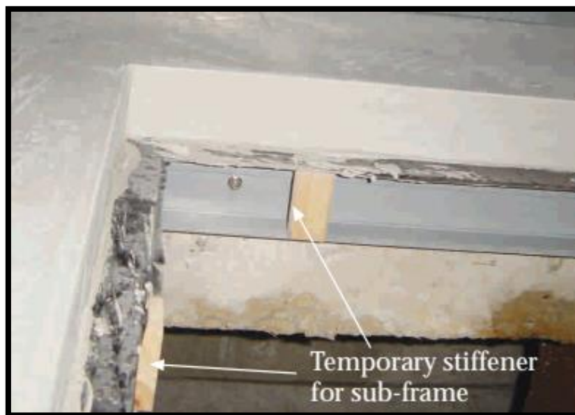
Installing temporary stiffener for sub-frame
