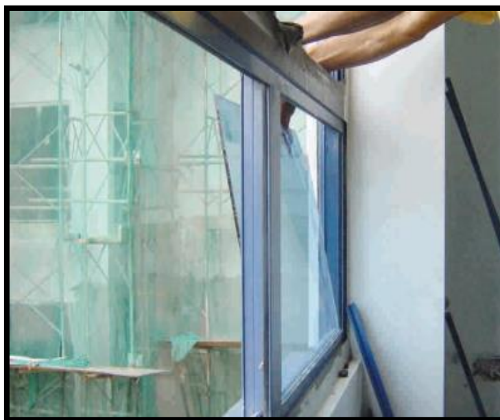
Window Glass Installation
