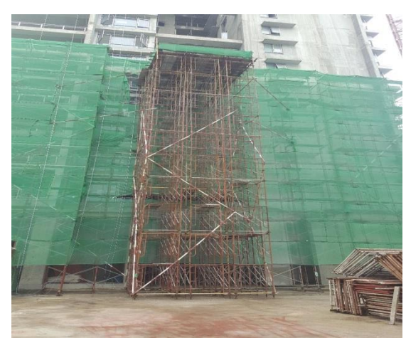
Material loading platform
