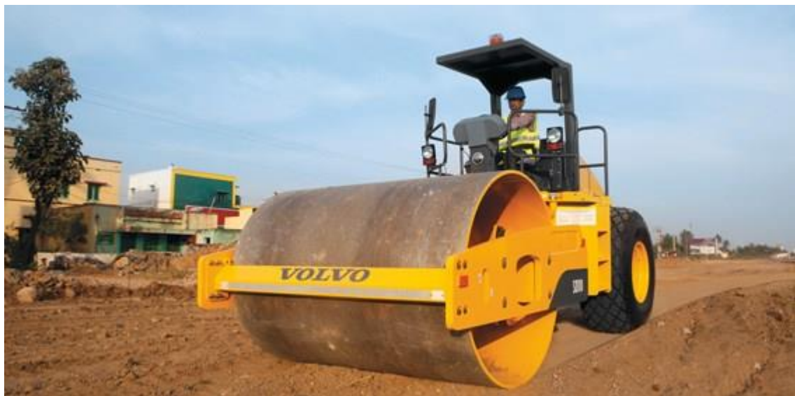
Compaction of soil
