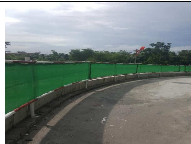
Hard barricade for edges protection
