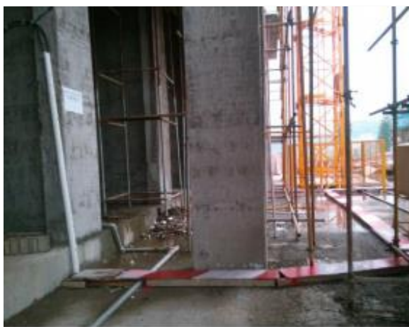
Floor wiring PVC sleeve fixed laying
