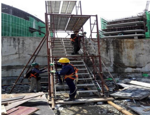
Access scaffold for car-park roof.
