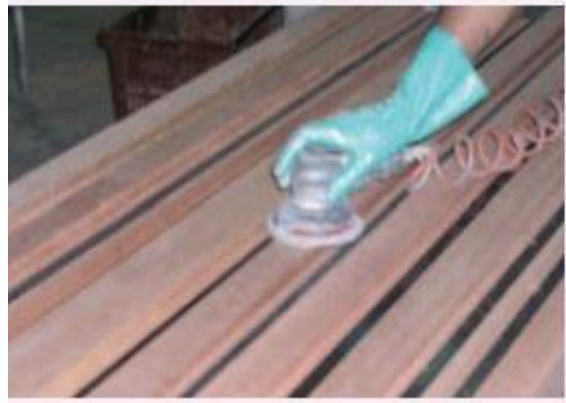
Sanding/grinding/skim coating Followed by rinsing with clean Water and wiping dry
