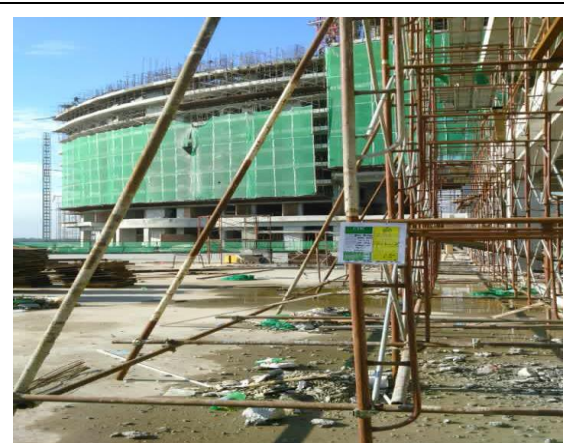
External scaffold on 1 st level tagged
