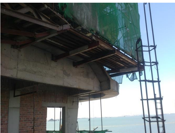
Cantilever supports for scaffold
