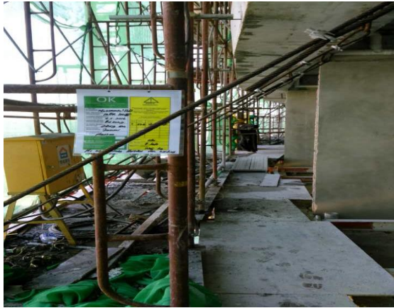
Cantilever external scaffold tagged.
