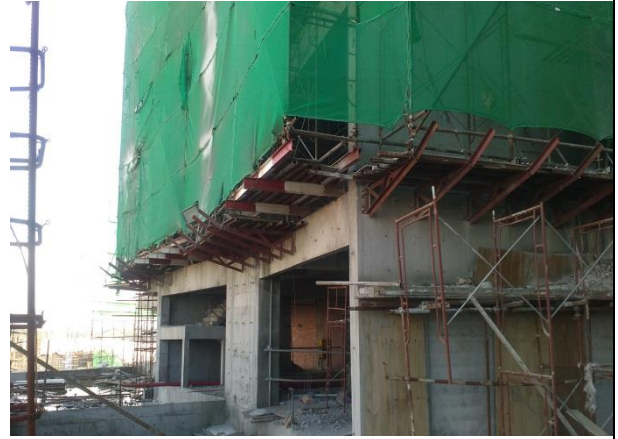
Cantilever supports for scaffold
