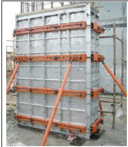
Aluminium formwork bracing
