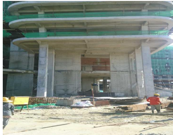
Dismantled cantilever scaffold and install safety railing.
