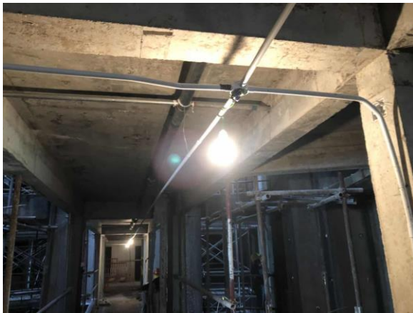
Temporary wiring at site
