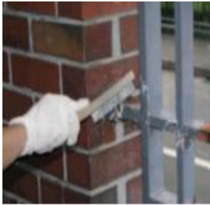
Manual cleaning by chipping, scraping and/or wire brushing
