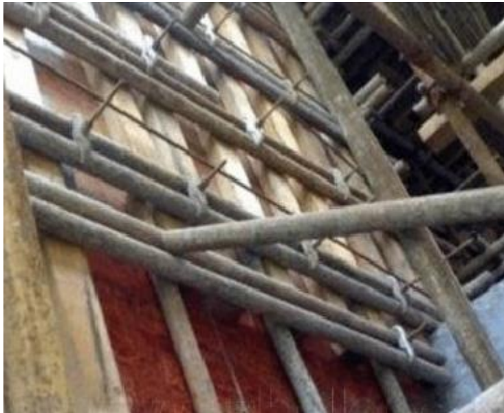
Shear wall template support
