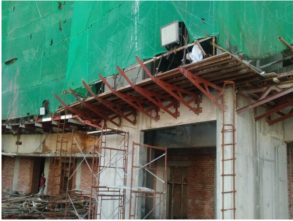
Side view of Cantilever supports for scaffold
