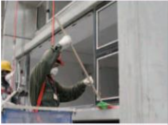
To remove foreign and unstable matters such as construction soot, concrete/cement splashes.
