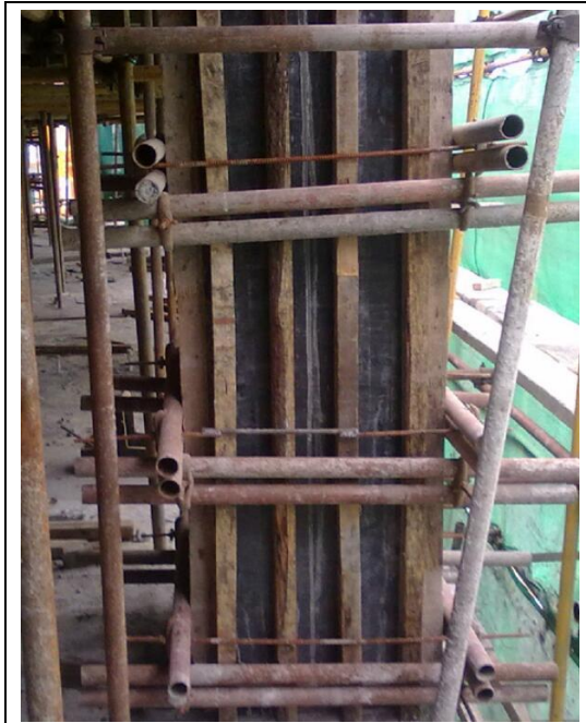
Rectangular column template support
