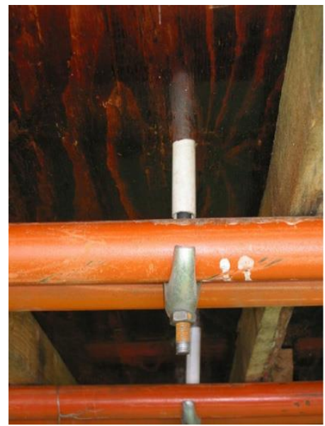
Split bolt wearing a PVC tube
