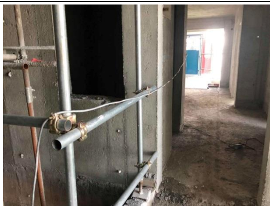
Electrical cable hanging to avoid soaking in the water and tripping hazard
