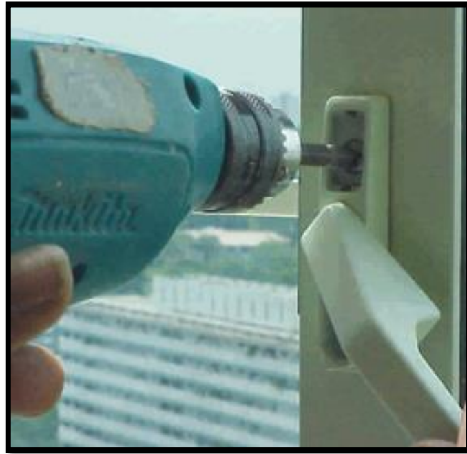
Fixing of handles
