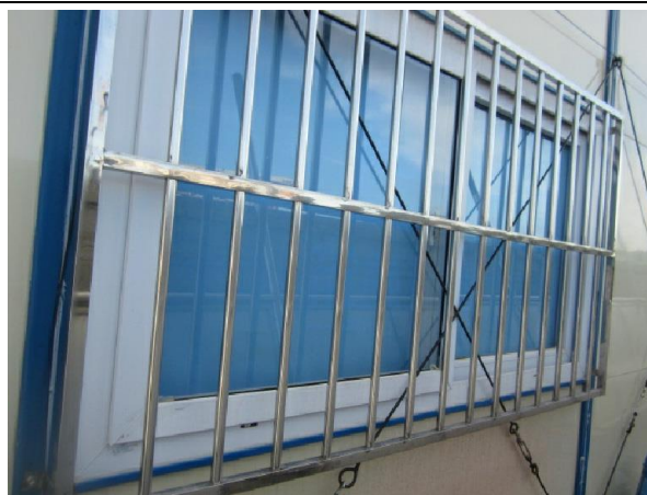
Stainless steel window grill (Recommendation)
