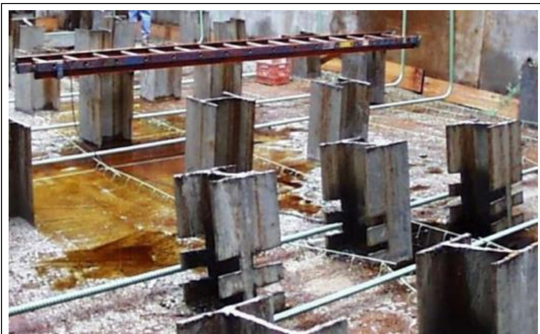
Example of Unacceptable Notches Cut into Piles
