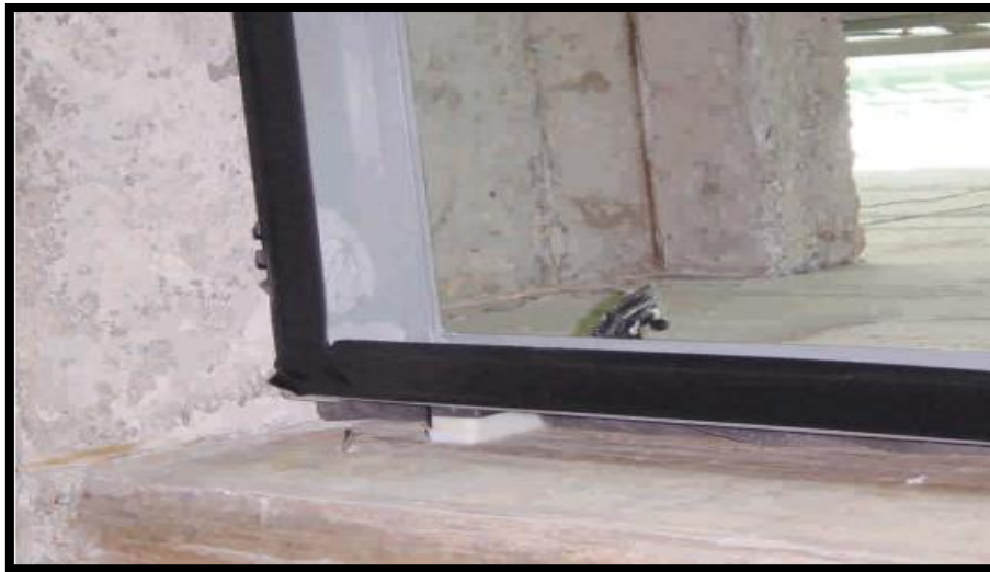
Positioning of sub-frame using ride up blocks or aluminum shin plates
