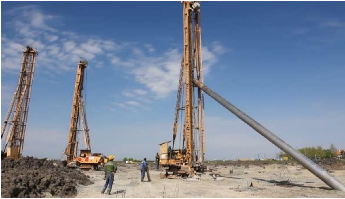
Moving rig on stable floor
