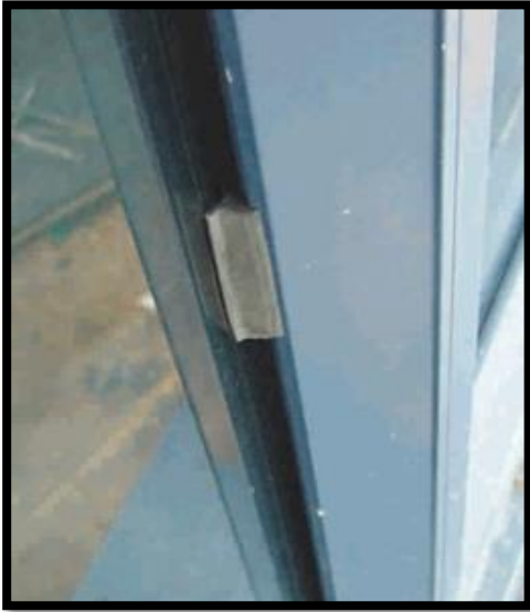
Insertion of spacer blocks
