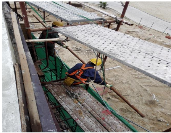
Installed horizontal bracing for scaffold
