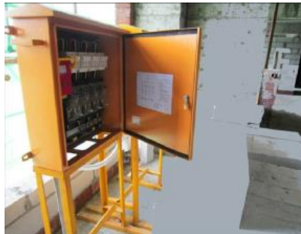
Temporary DB Box for each floor
