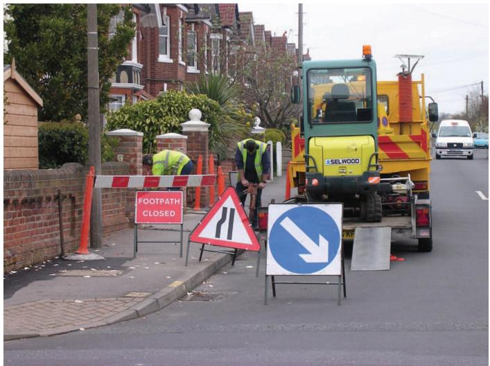
Figure 13. Working on or in close proximity to a highway or any other place where public vehicular traffic may cause danger to men at work, the working area shall be so barricaded and suitable warning signs and warning lights shall be set up to direct traffic away (Hughes, et al., 2008).
