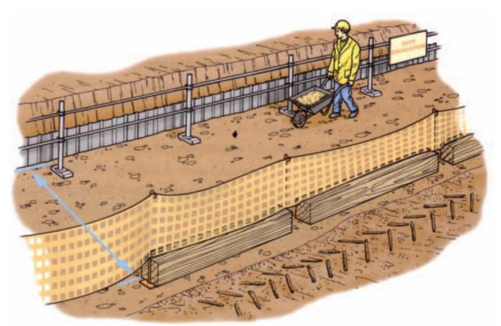
Figure 12. Vehicle protection at top of an excavation to prevent hazards associated with vehicle collision with its workers (Hughes, et al., 2008).
