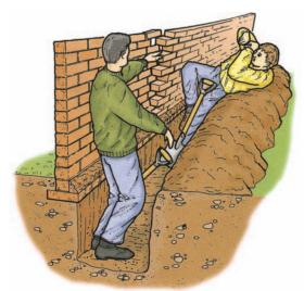
Figure 2. Stability of structures adjoining or over areas to be excavated must be protected (Hughes, et al., 2008). Where there is any question of stability of structures adjoining or over areas to be excavated, such structures shall be supported where necessary by underpinning, sheet piling, shoring, bracing or other means made or erected according to the design of a Professional Engineer to prevent injury to any person (FMA, 2014).
